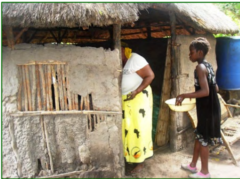
Below: Kamwengo brings the 'glue' in a bowl. You can see where the plaster has fallen off the wall (this is a cooking hut). The new plaster will be applied over the underlying structure.
